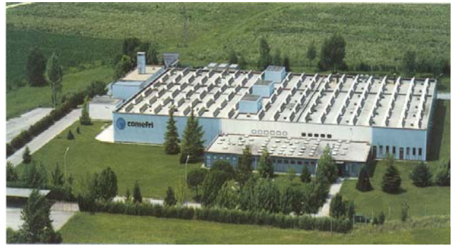
COMEFRI SpA factory at Arterga (UD) – Italy with 6.300 m 2 workshop. Production of industrial fans and special executions.
